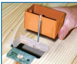
Install clip over subfloor.
