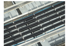
Large power cables
