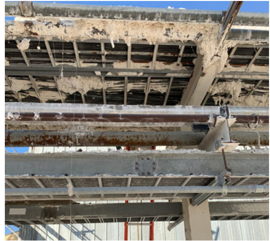
Chemical and atmospheric corrosion on a cable tray installation at a paper mill
