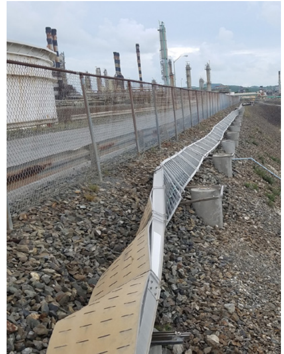
Cable tray damage due to high winds
