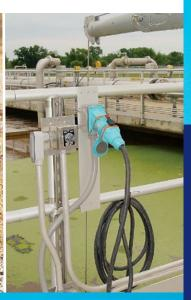
Switch-rated plugs & receptacles allow mixers to be connected and disconnected safely with plug-and-play simplicity. Mechanics can easily replace or service the mixers without the need for cumbersome PPE (personal protective equipment) because the switch-rated plugs and receptacles meet NFPA 70E's 'Normal Operation' definition.
