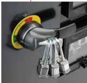
EXTERNAL MAINS BREAKER ACTUATION
