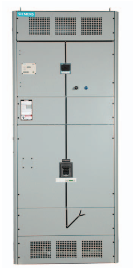
Switchboard with Sm@rt DAS
