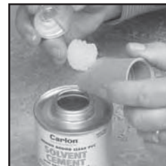
Apply a uniform coat of cement.
