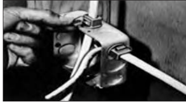
Snap captive locking wedge into connector's cavity.
